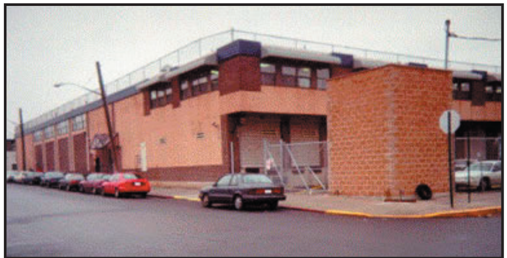
Queens Private Correctional Facility, 182-22 150th Ave.
